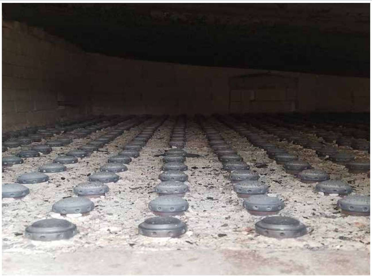
Figure 2: Combustion chamber of fluidized bed boiler
